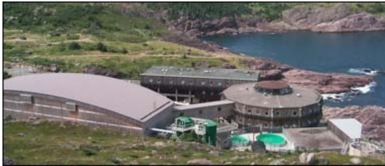
Figure 22: The Ocean Sciences Centre and it’s Aquaculture Research and Development Facility (ARDF) to the far left.
